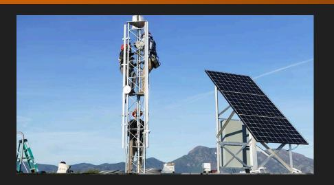
UNR Seismological Program for remote mountain top cameras for fire detection and monitoring.
